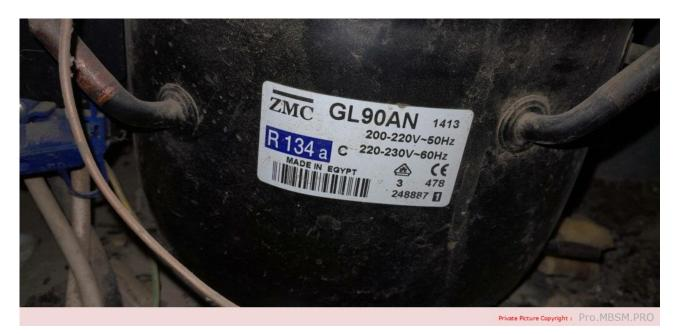
Pro.mbsm.pro, Compressor, R134a, Cubigel, ZEM-ACC, GL90 AA , 1/4 hp++, R134A
